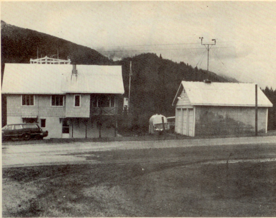
Mullan Pass (Idaho) FSS, which FAA said is one of only two remaining FSSs in the "lower 48" not located on an airport, would be decommissioned under proposed reorganization plan. Zuni (N.M.) FSS, located on an Indian reservation, is the other facility, according to FAA officials. It too would be shut down. Photo courtesy of Mullan Pass FSS
