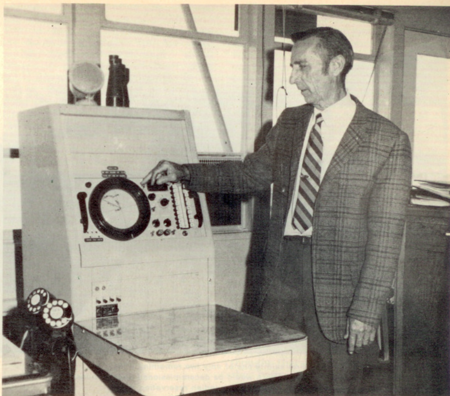
R. J. Christiansen, chief, Cedar City (Utah) FSS, explains operation of direction-finding (DF) equipment used in assisting pilots who become disoriented while in flight. Located on the Cedar City Municipal Airport, the FSS would become one of 155 full-time Level IV FSSs under updating program. All Level IV FSSs would be equipped with DFs under the program. Photo courtesy of Cedar City FSS
